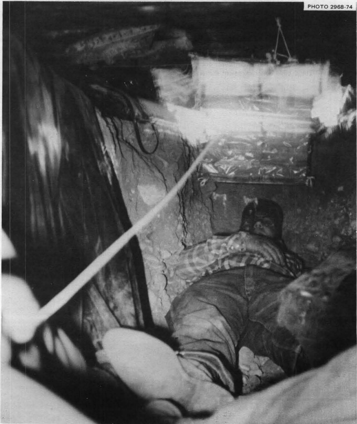
Fig. 6.16. A 17 × 19 in. KAP being used to pump about 100 cubic feet per minute through a Car-Over-Trench Shelter, and out through the 110 square inch exhaust opening. Especially during hot, sunny weather, temperatures inside a Car-Over-Trench Shelter would become intolerable without adequate forced ventilation.
